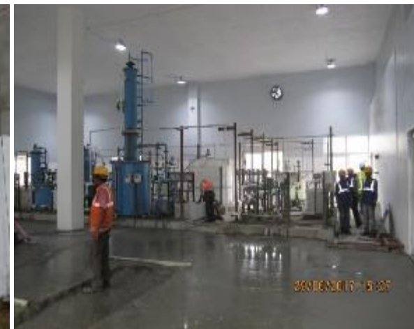
Demineralization Water Treatment Plant
