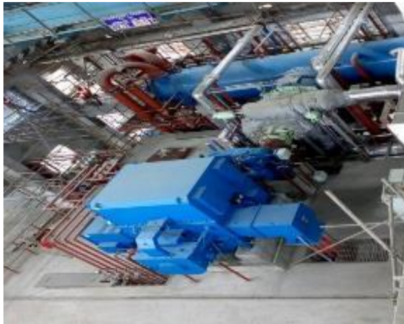
Steam Turbine Generator (STG)
